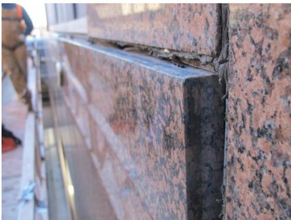
*Poor anchorage leads to 400-lb. granite facade panel breaking loose from high-rise building.*
