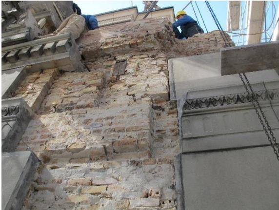
*Displacement of limestone veneer due to corroded anchorages required its careful removal and reinstallation.*
